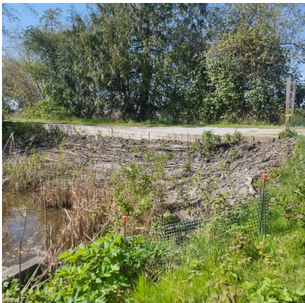
Completed wattle fence
