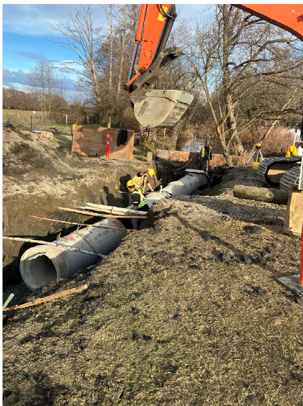
Replacing the culvert under the road by the washrooms.
