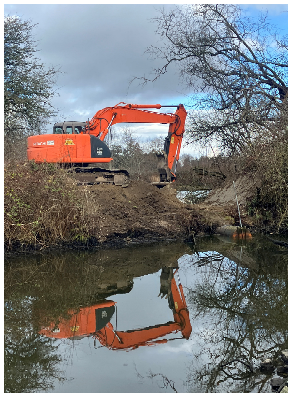
Digging out the old Fuller Slough water control.
