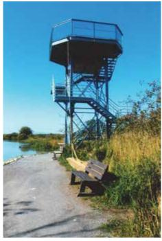
The blue metal tower was built in 1981 in the West Field to replace the wooden tower. The metal was salvaged from scaffolding used in the construction of the atriums of Lansdowne Shopping Center in Richmond.
